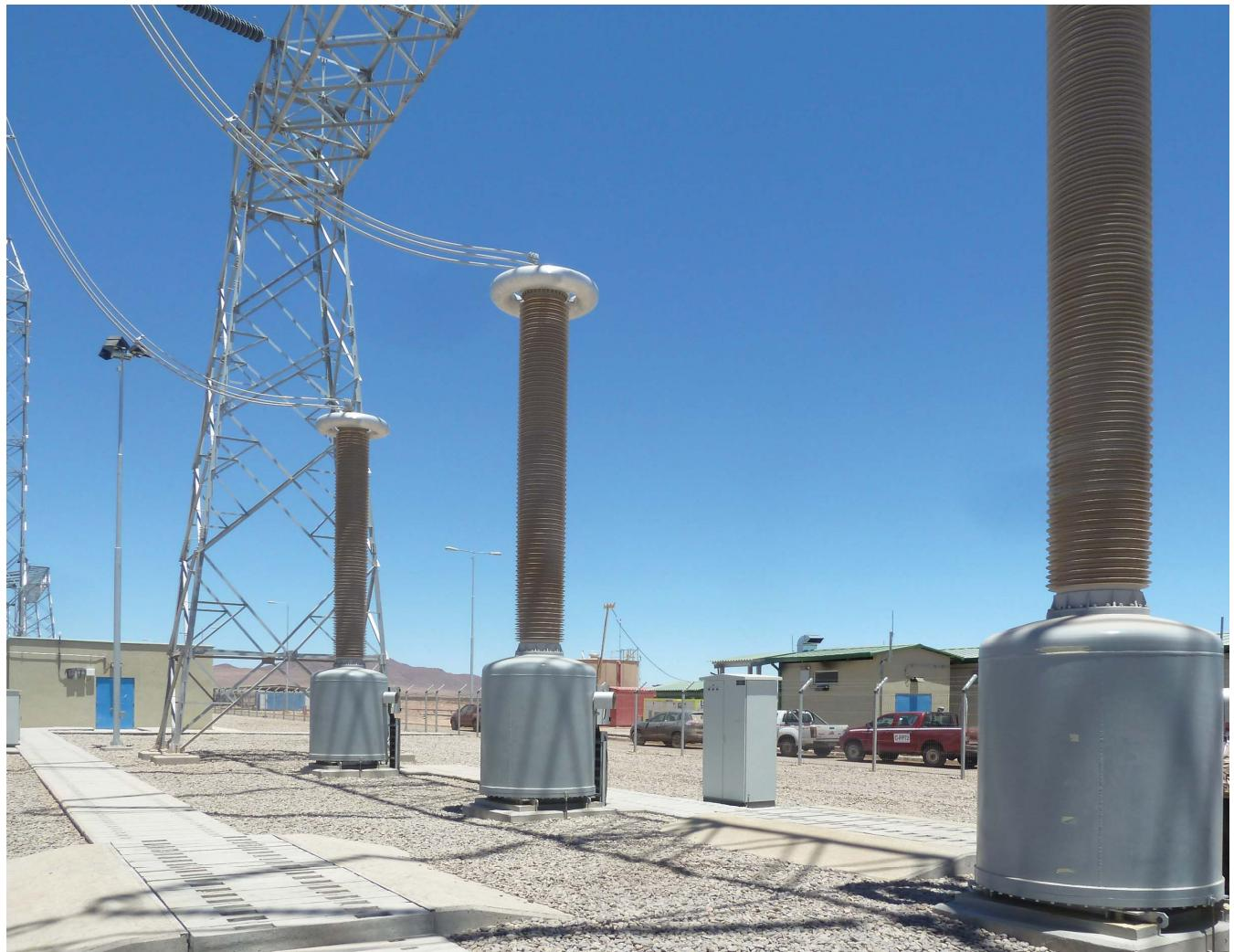
Power Voltage Transformers (PVT) also known as Station Service Voltage Transformers (SSVT) are used to supply Low Voltage power directly from a High Voltage line up to 550 kV. Located within the own substation they can provide power up to 333 kVA per phase in a reliable and cost-effective way. They offer a wide range of applications, but they excel when substation auxiliary service power supply is needed in remote areas, making them an ideal solution for Renewable Energy substations.
