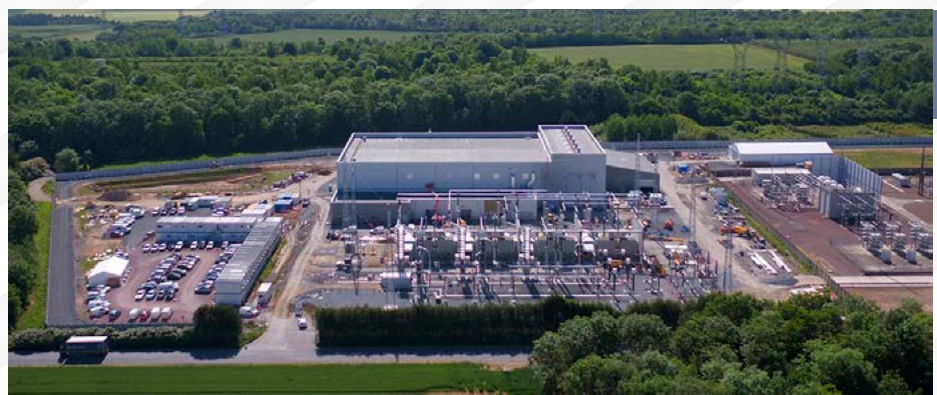
Substation at the French end of the Channel for the France-England interconnection
